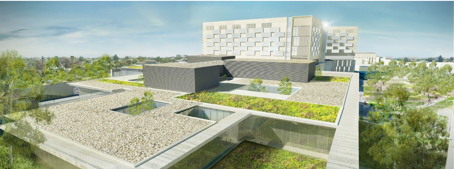
Image of the new Bendigo hospital, showing the green roof and landscaping.
