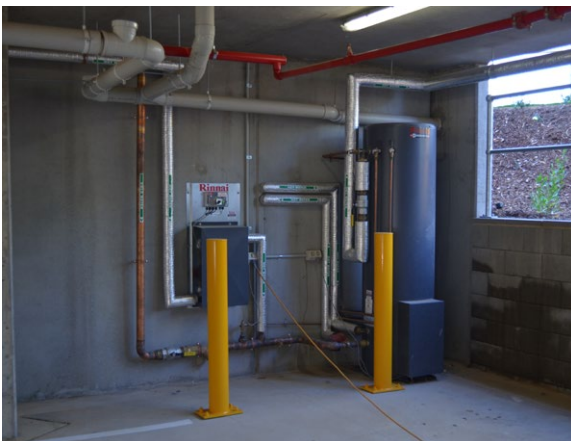
The hot water systems installed at Atkins Street complex, showing the instantaneous units (top) and storage tank and recirculating pump (bottom).
