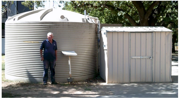
Leading hand Gardener Bob Ermel in front of the garden irrigation tank.
